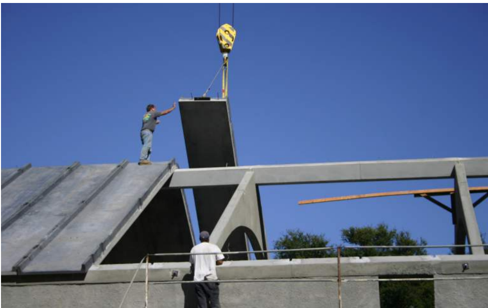
Installing the roof panels
