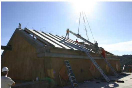
Integral Solar Roof installation
