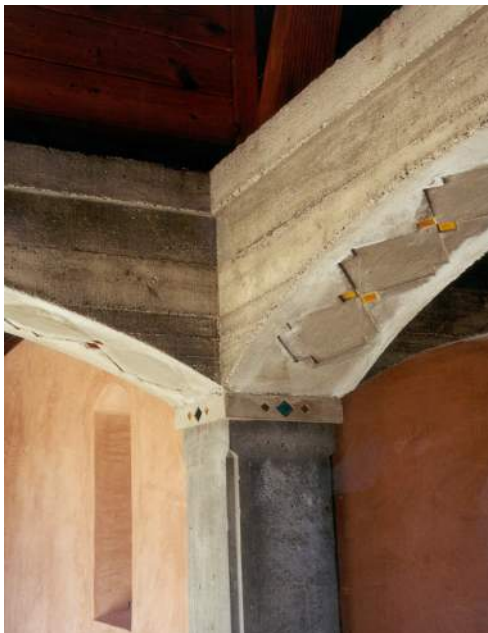
Cast Concrete columns and Beams
