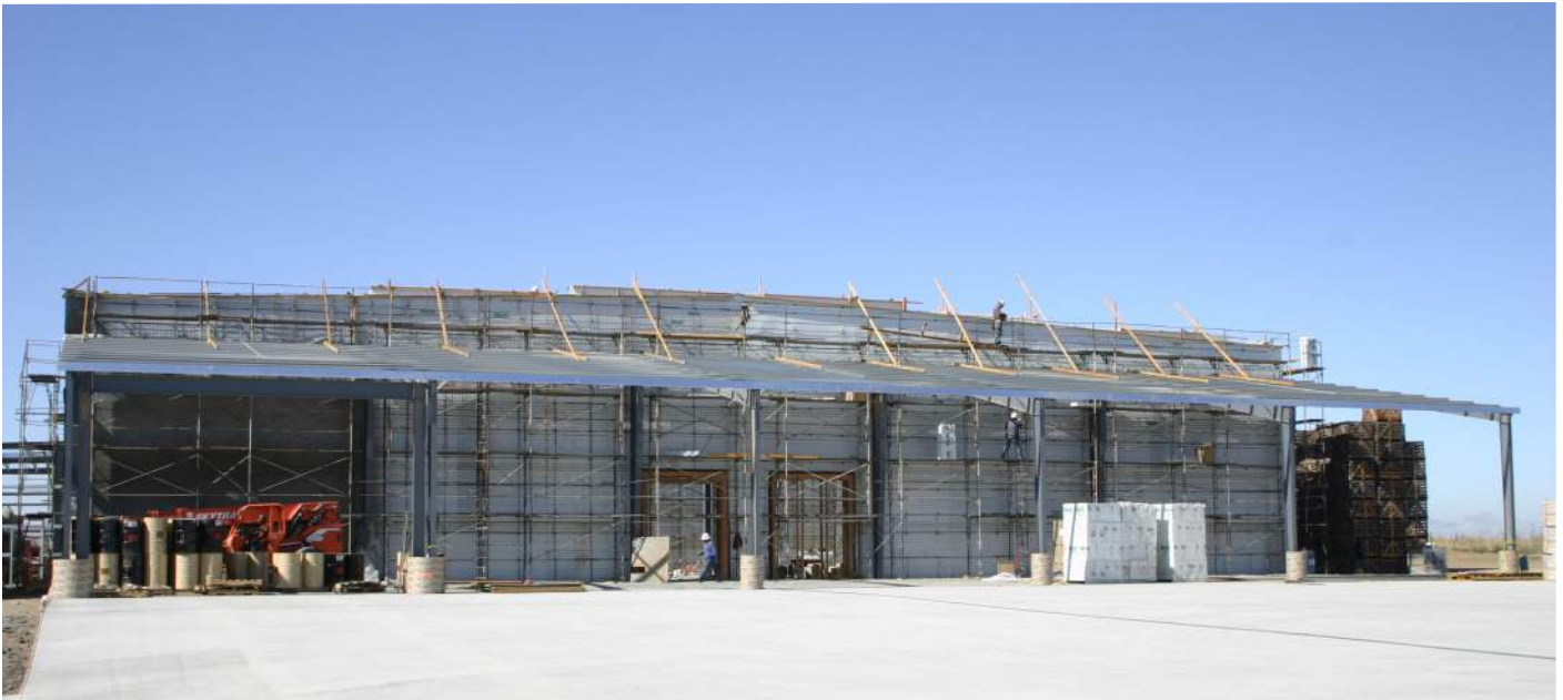
Cold Storage bldg. under construction
