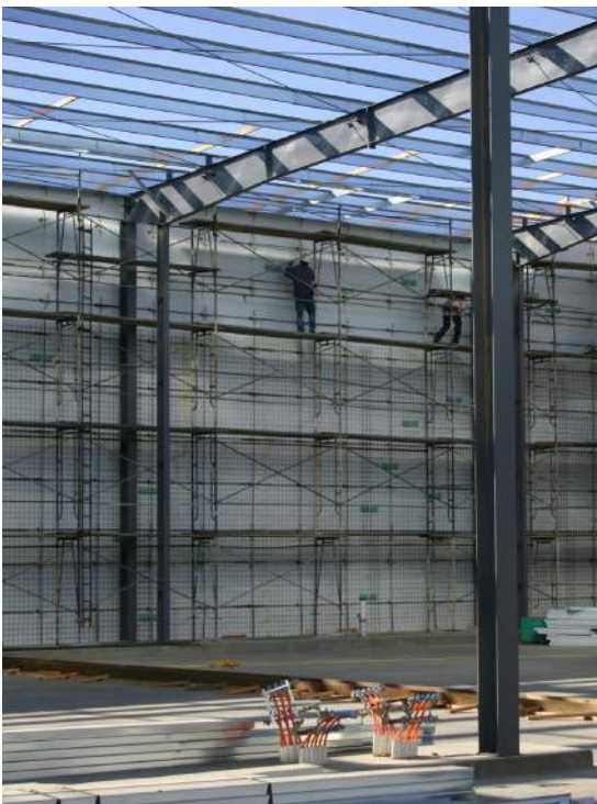
Cold Storage, under construction
