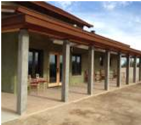
Western covered arcade
