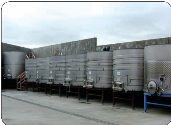
Outdoor Tanks at Laird Family Estates, Napa
