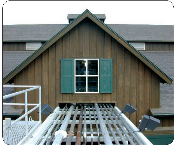
The fermentation building at this facility was a PRE-ENGINEERED METAL BUILDING with wood exterior.
